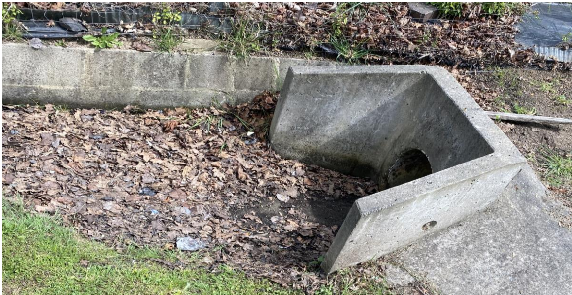
Figure 5.1.1: Existing Headwall (Site Visit, 2023)
